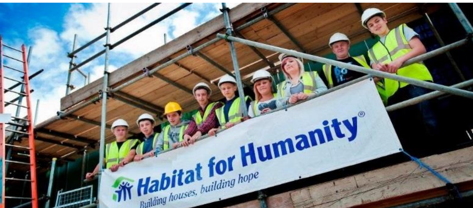
Trainees working on a Habitat for Humanity GB (Homes) project in Banbury.
