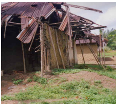
House in disrepair as a result of armed conflict.
