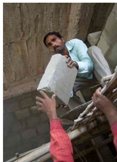
Top: Community center under construction.
