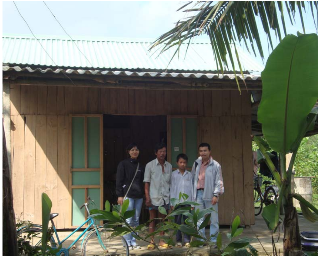
Right: A Vietnamese family in front of their repaired home.
