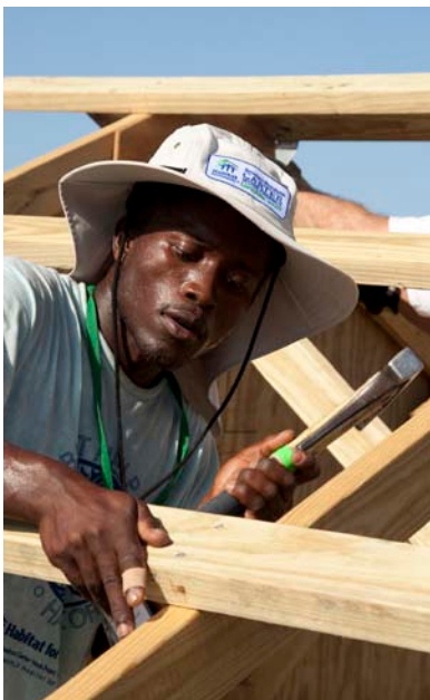
Beneficiary works on the roof of his future home.
