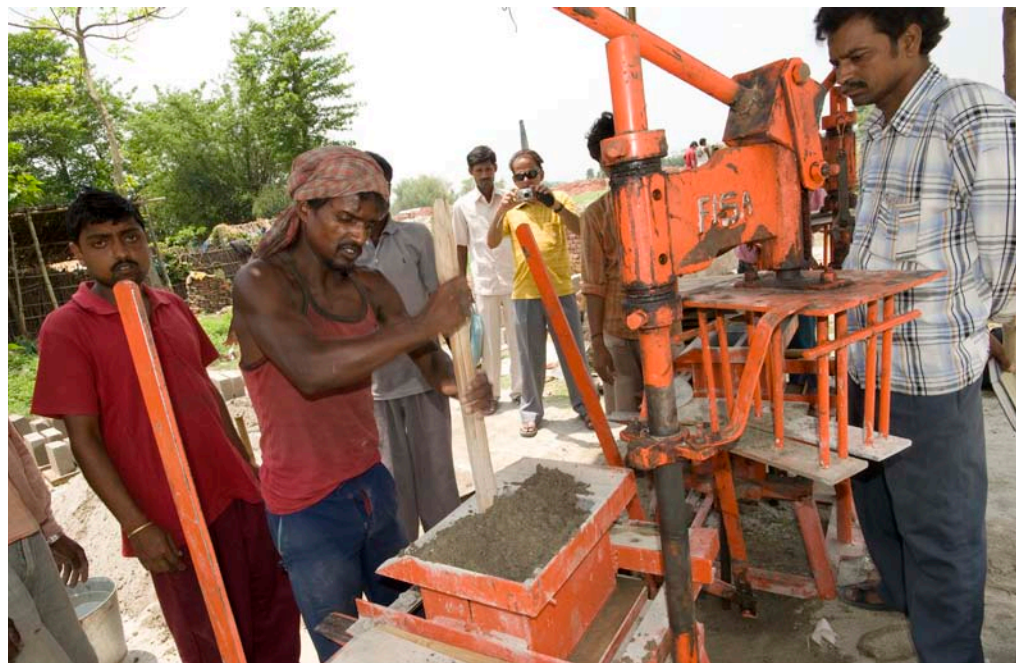
Right: Homeowner partners made bricks for their houses.
