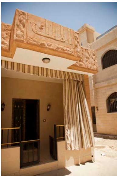
The Bazzi family's home was rebuilt with help from Habitat Lebanon.
