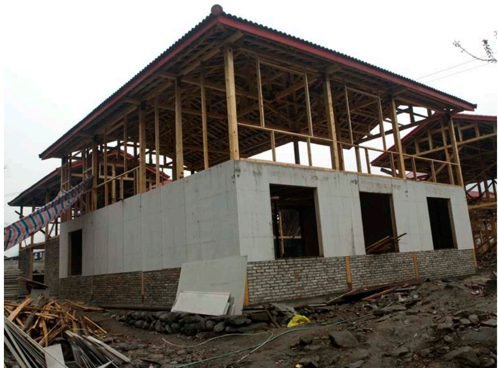
Right: A two-story housing solution under construction.
