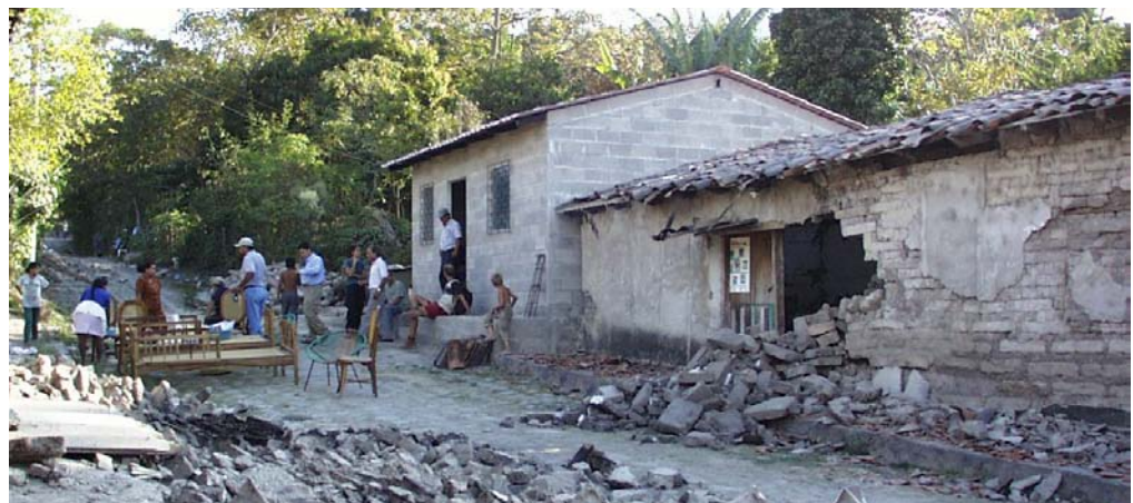
Right: A Habitat home stands amid damaged houses.
