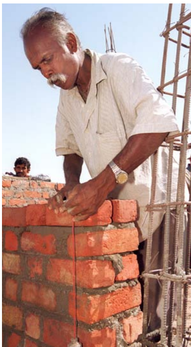
Local contractor checks progress on house construction in Khumbariya village.
