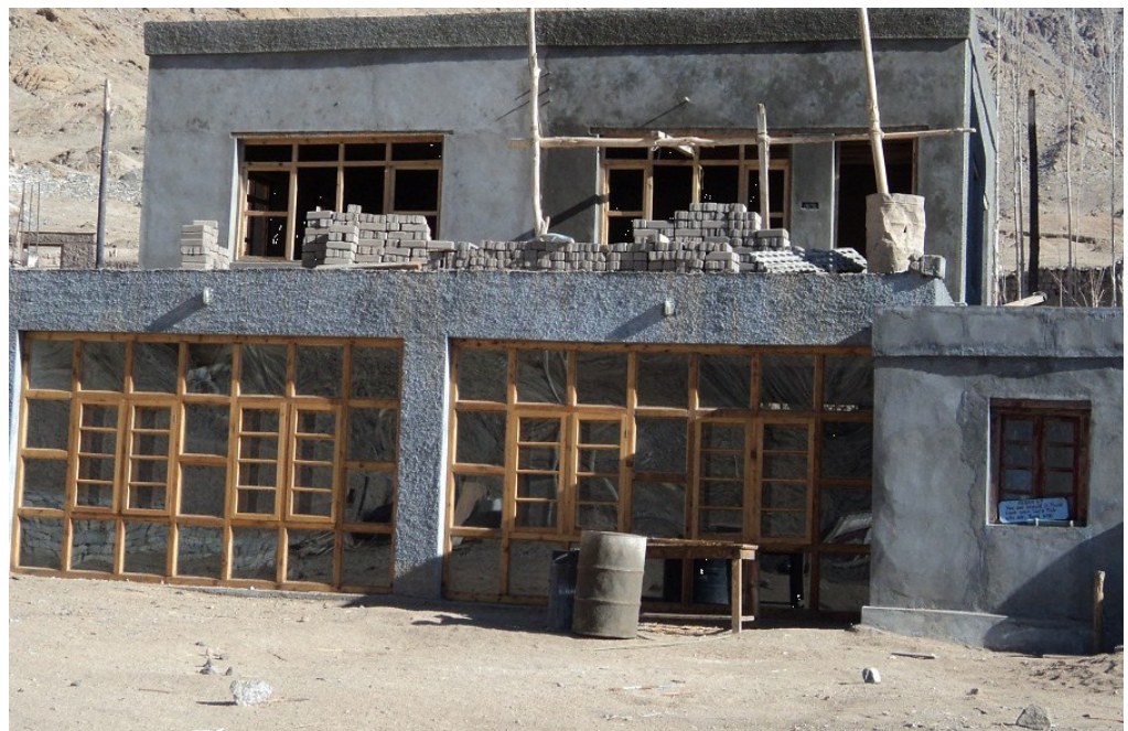
Right: House near completion.
