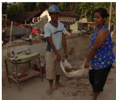
Family clears foundation to build temporary shelter.
