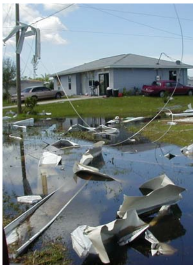
Hurricane Charley damage in Charlotte County, Florida, was severe.
