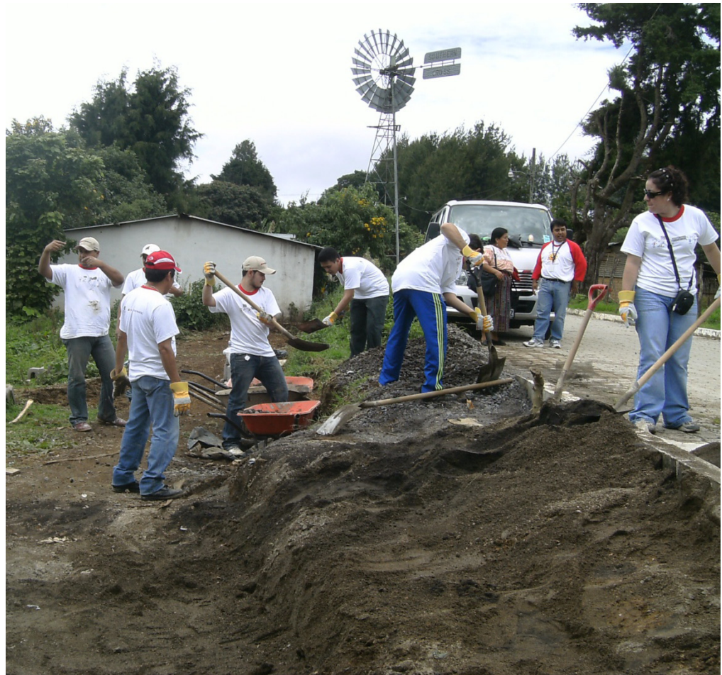
Right: Volunteers start a new home site in Guatemala.
