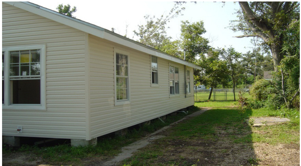
Right: A Katrina-affected home that was repaired in Bay St. Louis, Mississippi.
