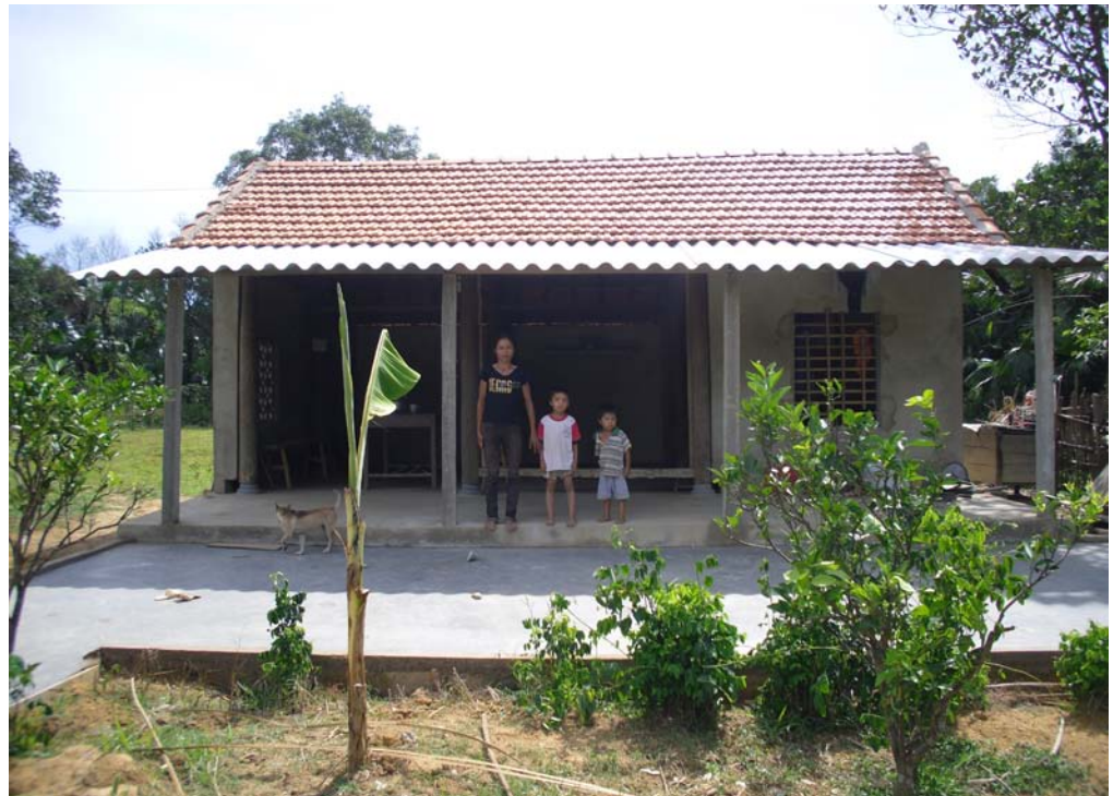
Right: Tran Thi Lai's new home.
