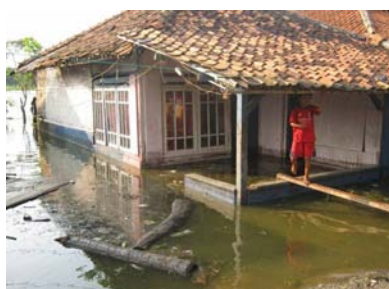
Home damaged by Karawang floods.
