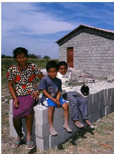
Family in front of their new Habitat home, under construction.
