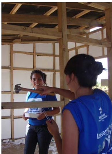
Habitat staff work on a house in Curepto, Chile.
