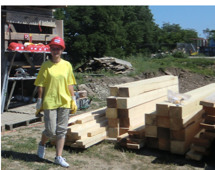
Christina on site, helping to build her new home
