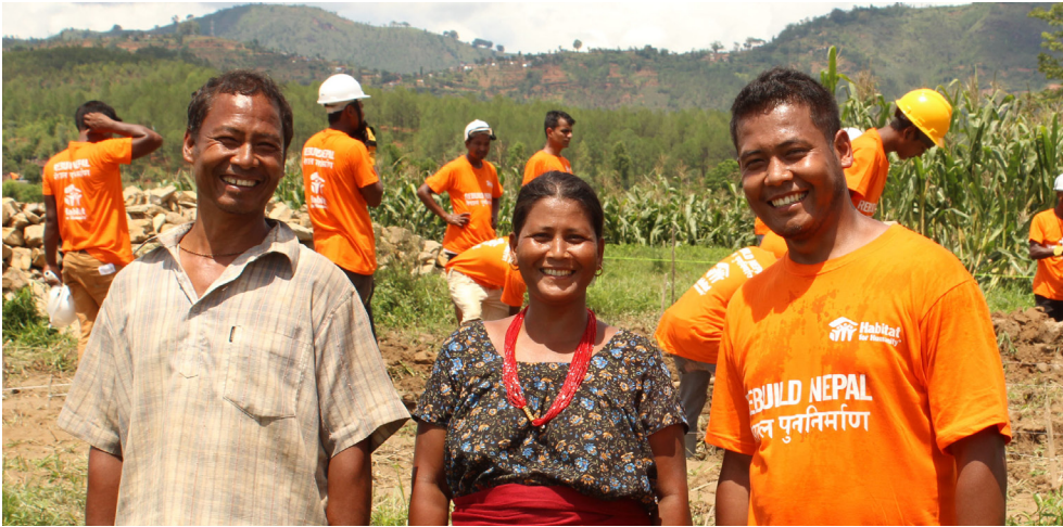
Ranuki Danuwar (center), with her husband Kansa (left) and son Simiraj (right), at the groundbreaking for the construction of their new home in Pipaltar village, Kavre district, the first of permanent houses that Habitat will build as part of the earthquake response.
