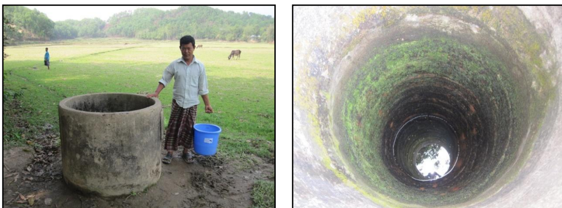
Figure 9: Community practice in Durgapur (Unprotected Dug well)
